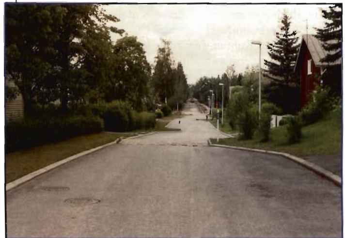
Traffic calming measures, such as the staggered narrowings and speed humps shown here in Kerava, Finland. These features have been effective in reducing motor vehicle speeds and enhancing safety.
