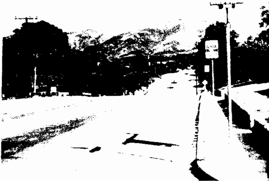
Figure 11: BI-DIRECTIONAL LANE (Santa Barbara, California) NOTE NON-STANDARD SIGNING, INDICATING LANE AND PART-TIME (During School Commute Hours) PARKING BAN
