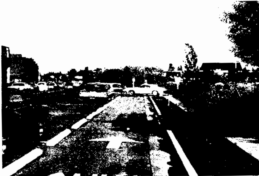
Figure 12: TYPICAL PROTECTED LANE (Davis, California) NOTE USE OF CONCRETE "PARKING LOT BUMPER BLOCKS" AS BARRIER
