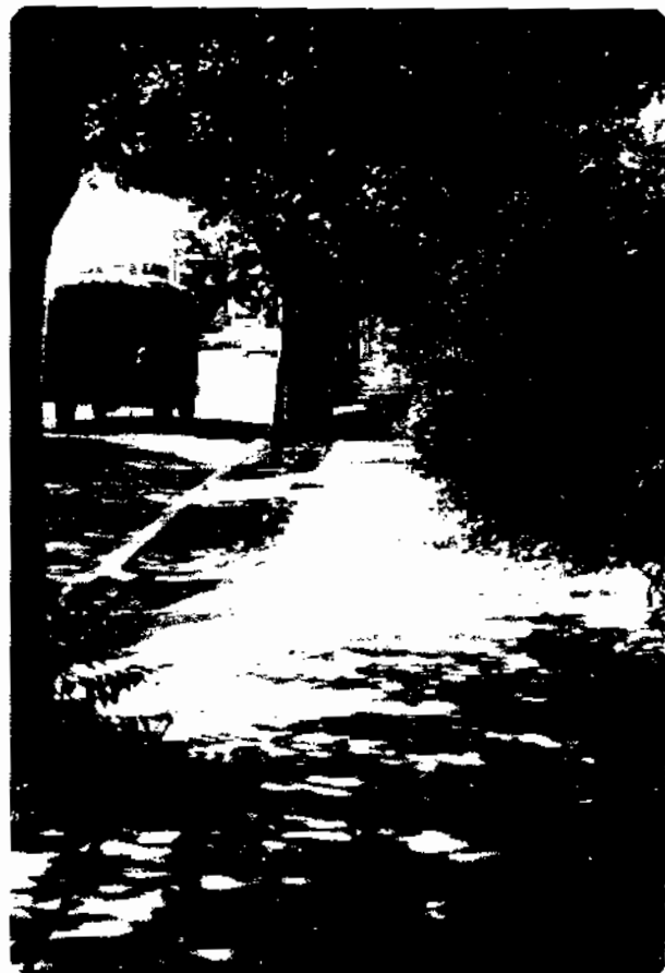
An uninviting sidewalk bikeway. Note shrubbery obscuring driveway view and reducing effective width of already narrow sidewalk
