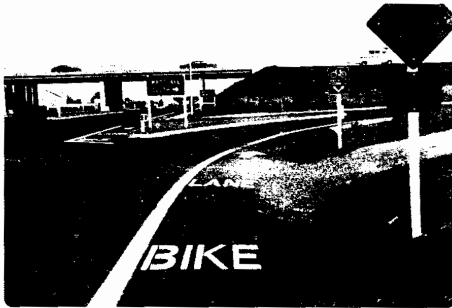
Figure 33: RIGHT ANGLE CROSSING OF INTERCHANGE RAMP. BETTER PAVEMENT MARKING OF CROSSING AREA AND BERMS TO POSITIVELY CHANNELIZE CYCLISTS INTO PROPER CROSSING ANGLE WOULD BE DESIRABLE
