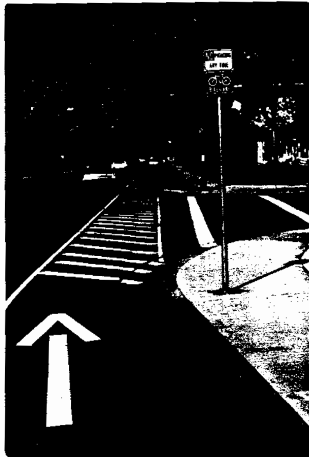
Figure 31: BIKEWAY MARKED THRU INTERSECTION WITH DIAGONAL LINES FOR ADDED VISIBILITY AND EMPHASIS (Cupertino, California)
