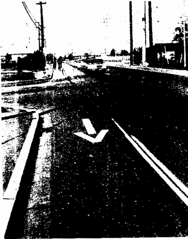
Figure 37: DIRECTIONAL ARROW USED AS BIKE LANE DESIGNATION MARKING. PROVIDES LITTLE INDICATION TO MOTORISTS OR CYCLISTS THAT THIS IS, IN FACT, A BIKE LANE
