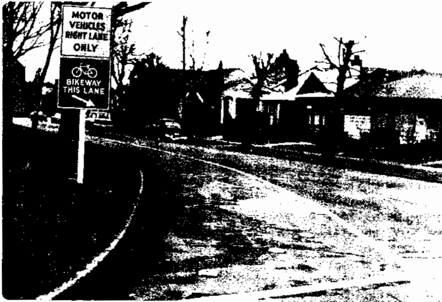
Figure 10: LEFT SIDE LANE POSITIONING ALONG WIDE MEDIAN (Seattle, Washington) NOTE SIGNING PAVEMENT STUDS TO FEND TURNING CARS OUT OF BIKE LANE
