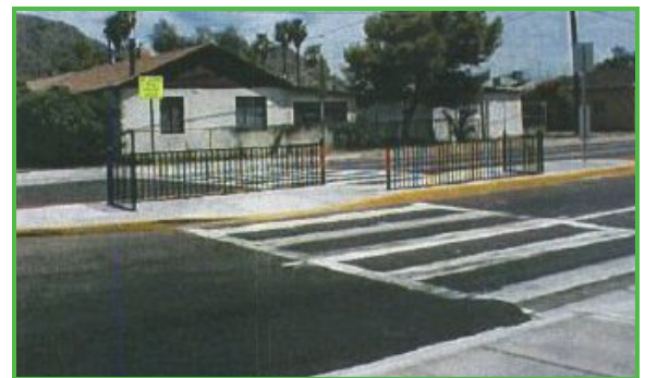
A staggered crosswalk installed for the program.
