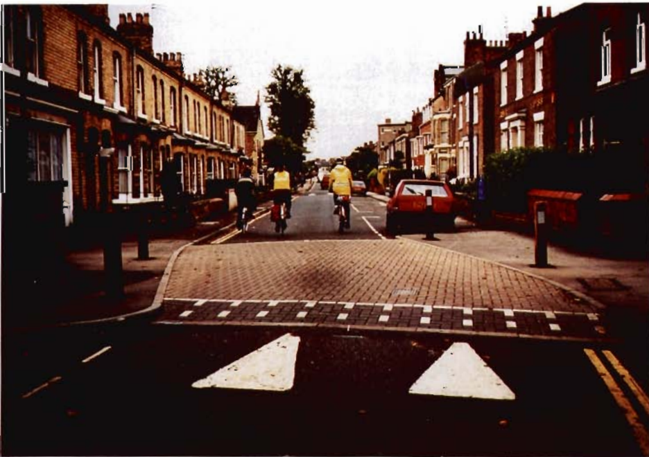
Figure 18. Speed humps slow traffic speeds on residential street in York, England.
