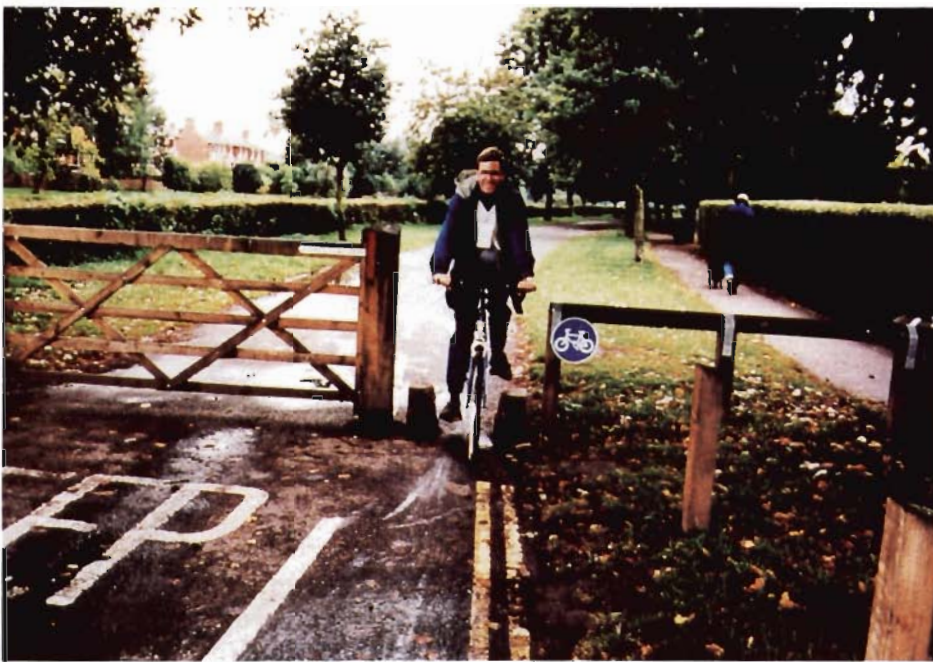
Figure 16. Entrance to bicycle trail is designed to restrict entry by motor vehicles.
