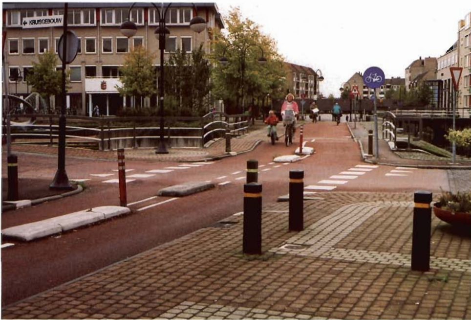
Figure 34. Intersection design in Houten gives priority to bicyclists and pedestrians over motor vehicles.
