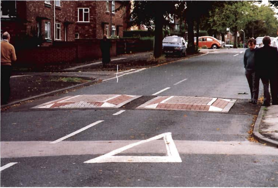
Figure 21. "Speed cushions" in use on a residential street in the English city of York.
