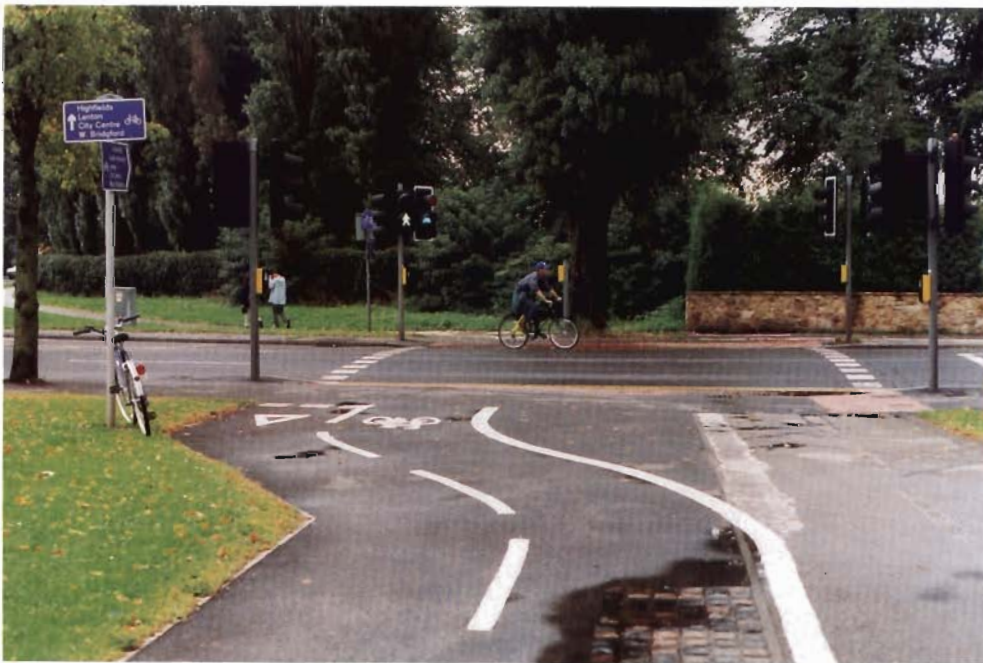
Figure 4. Toucan crossings in Great Britain provide separate pedestrian and bicyclist signals where trails cross roadways.
