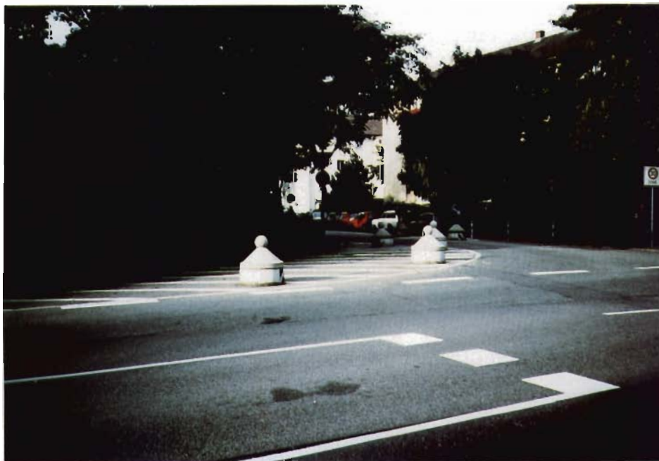
Figure 47. Concrete bollards are used in Freiburg for traffic calming.
