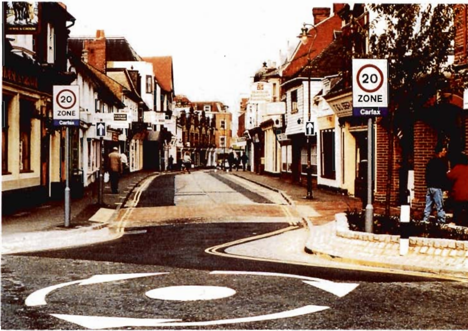
Figure 17. Networks of 20-mph zones in British neighborhoods often include signs, narrow streets, speed humps, or other measures. The combination of multiple measures on a neighborhoodwide basis is most effective.
