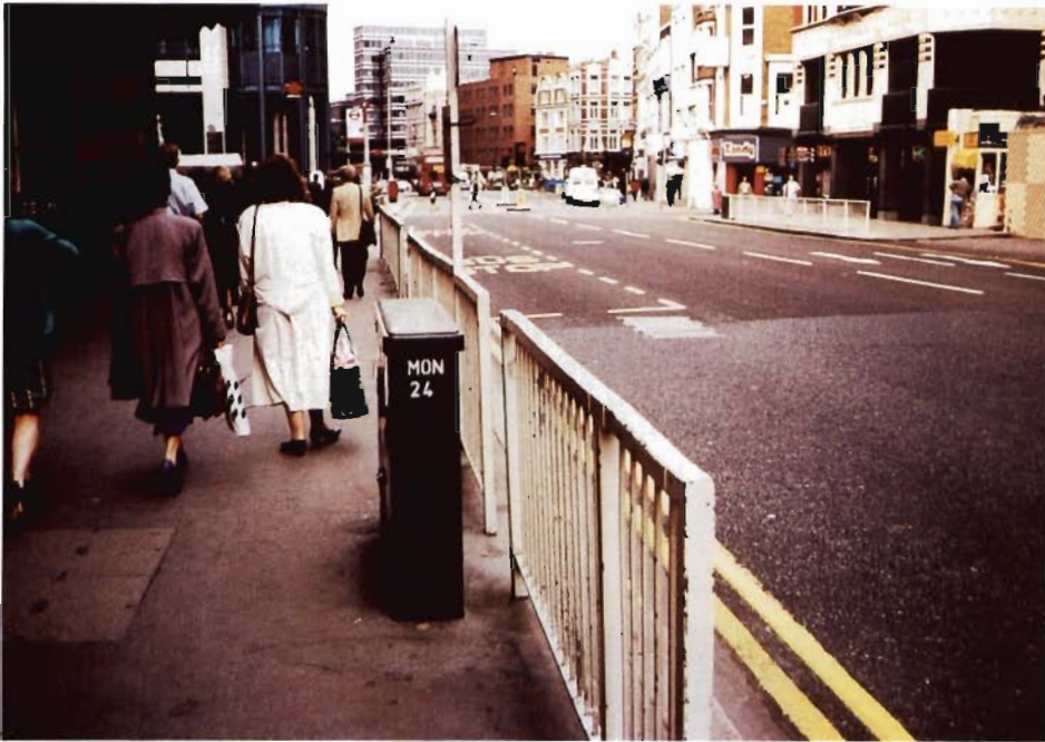
Figure 6. Pedestrian barriers (separators) are used extensively in London to channel pedestrians to preferred crossing locations.
