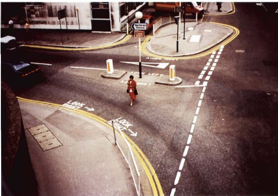
Figure 5. Pedestrian pavement messages and refuge islands.
