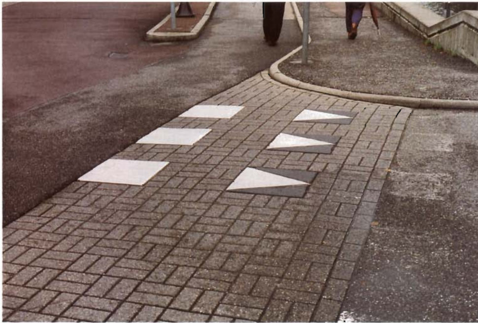
Figure 35. Triangular pavement marking shapes built into the pavement at this location indicate that motor vehicle traffic must yield to cyclists and pedestrians.
