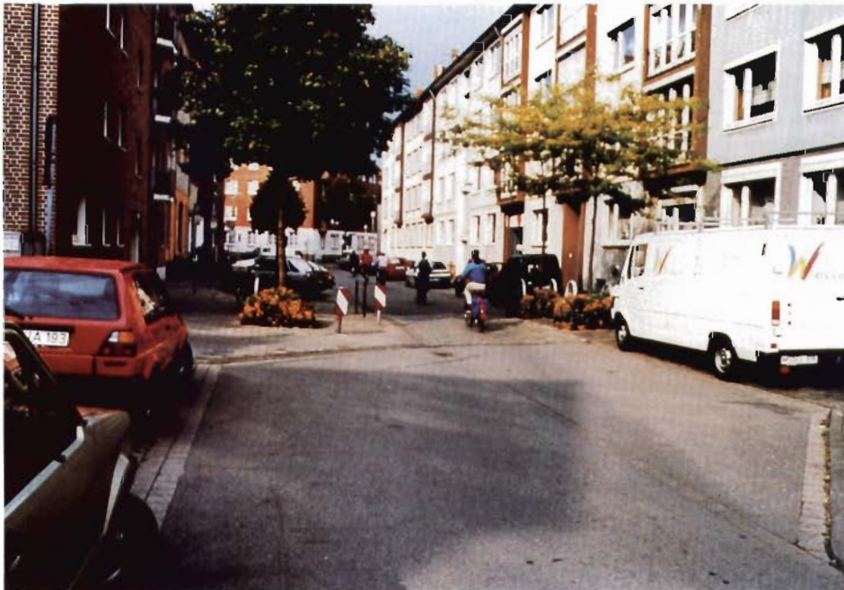
Figure 49. Example of a midblock narrowing in Germany to slow vehicle speeds.
