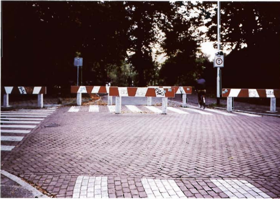
Figure 31. Barriers are used to block motor vehicles and allow bicyclists through traffic on this Dutch street.
