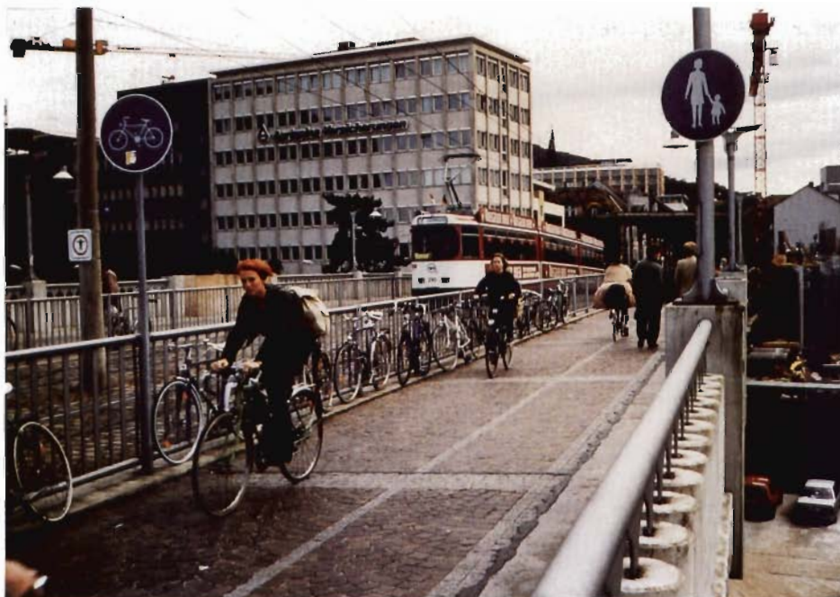
Figure 45. Pedestrian and bicyclist bridge near Freiburg rail station.
