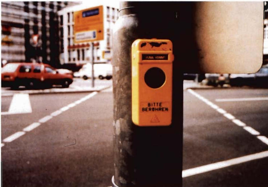
Figure 37. Pedestrian pushbutton device gives feedback “SIGNAL KOMMT” (signal is coming) to waiting pedestrians.
