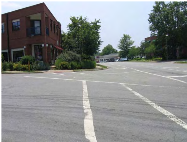
Figure 49. Wide expanse of pavement with only 'paint' for refuge. Two legs of the intersection lack pedestrian walk signals.
