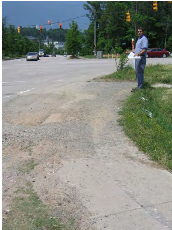
Figure 73. There is no curb and poor delineation between the road and pedestrian pathway at south side of Raleigh Rd and Barbee Chapel E.
