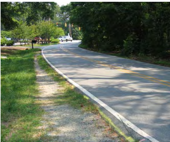
Figure 74. View of of Finley Golf Course Rd on approach to Raleigh Rd and adjacent path.
