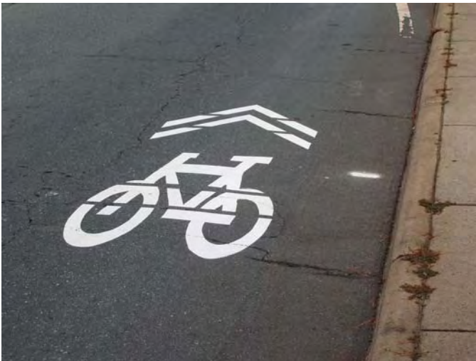
Figure 42. Sharrow (shared lane) pavement marking, as currently being evaluated on Martin Luther King Jr Blvd in Chapel Hill.
