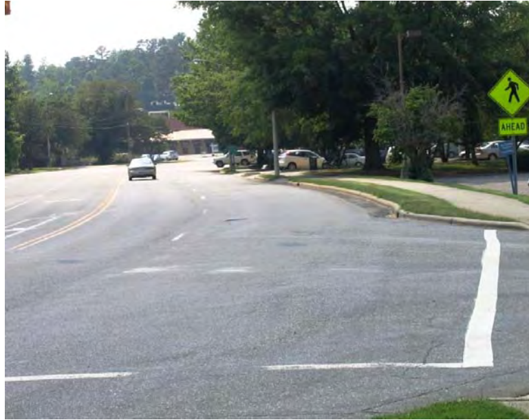
Figure 54. Estes Dr showing part of intersection with Willow Dr (and missing crosswalks) and views of driveways west and area where pedestrians often cross midblock.
