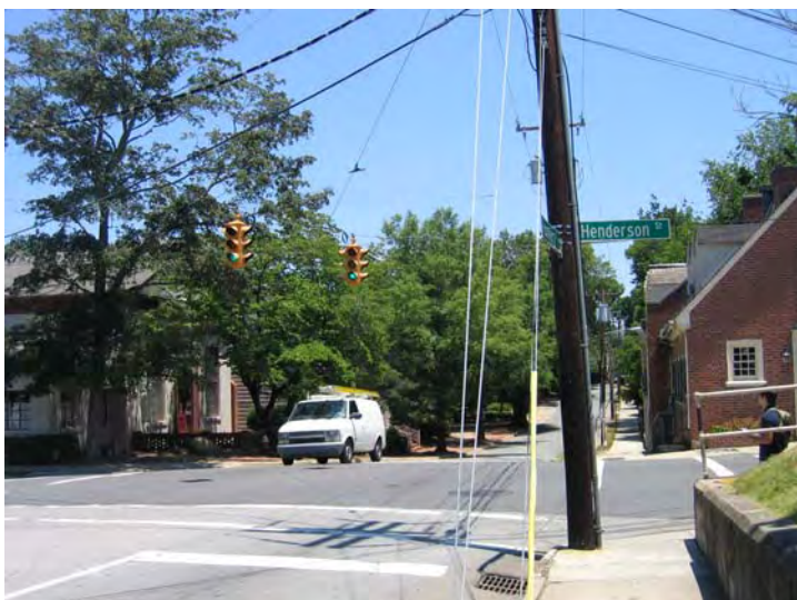
Figure 25. Pedestrian signals are lacking; utility pole narrows useable space and may obstruct visibility; curb is nearly level with the street, with no detectable ramp for pedestrians with disabilities at the corner of Rosemary and Henderson Sts.
