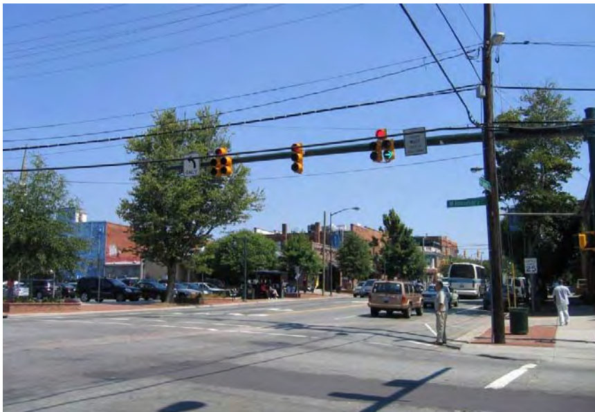
Figure 24. Utility lines obscure regulatory signs and traffic signals; pavement markings are worn and paved over at Columbia and Franklin St.
