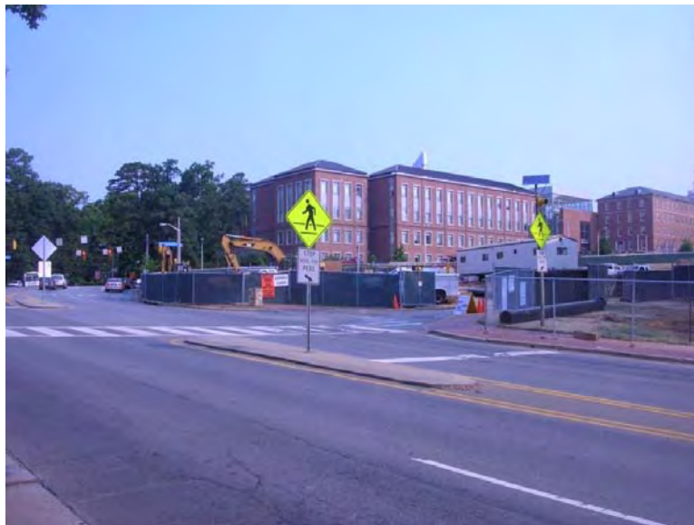
Figure 62. Closing sidewalks may result in extra roadway crossings and increased exposure for pedestrians. (Photo by Charlie Zegeer)
