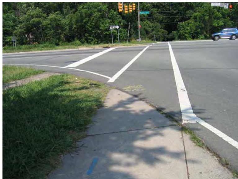
Figure 55. A lack of a curb and wide turn radius may allow high-speed turns from southbound Fordham onto Estes.
