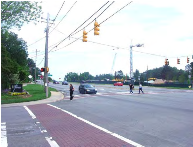
Figure 70. Advance stop bars and reallocation of lane uses could reduce the risk of multiple threat collisions and free up space for bicyclists and transit.
