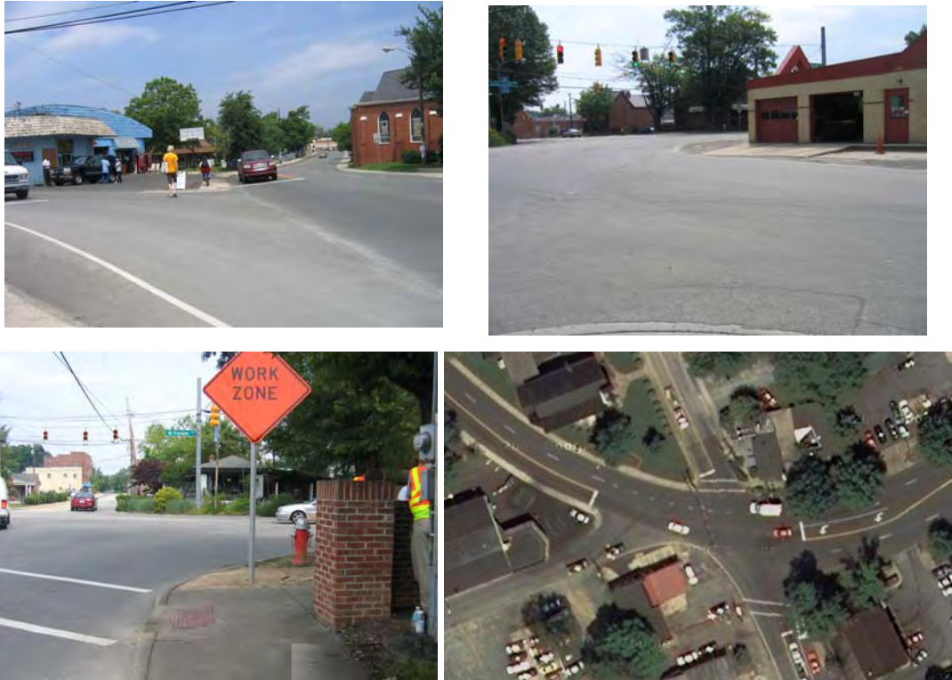
Figure 39. The multi-leg intersection of Franklin, Main, Merritt Mill, and Brewer provides a large expanse of unmarked pavement for pedestrians, cyclists, and motorists to navigate. (Lower right image from Google Imagery © 2008 U.S. Geological Survey.)
