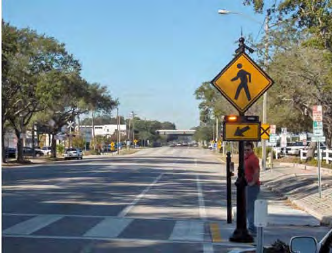
Figure 28. The rapid-flash beacon has also been evaluated for multi-lane crosswalks and has achieved a high rate of yielding over a sustained time period (Van Houten and Malenfant, n.d. Image from Van Houten and Malenfant).
