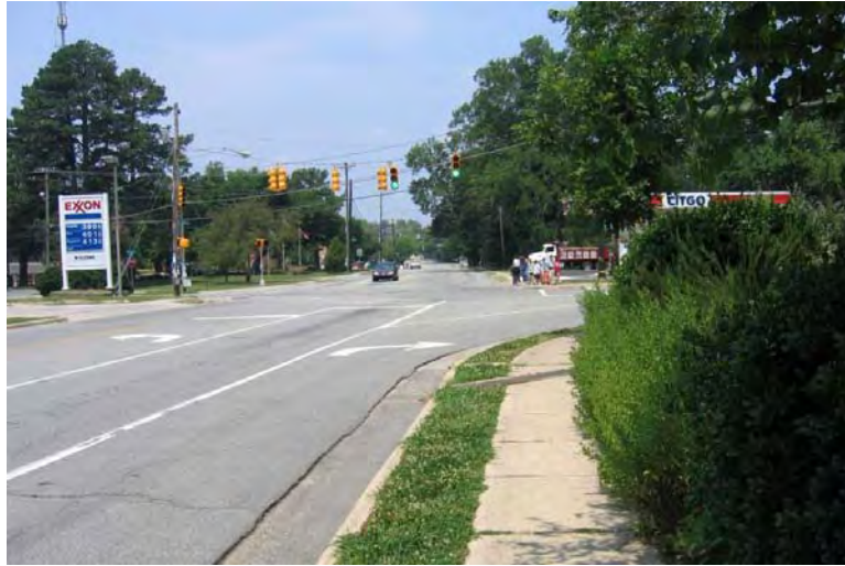
Figure 50. Crosswalks across right-turn flow lanes should be prior to the curve of the turn. On NW-bound W Main at W Weaver, shrubbery also obscures the view of the crosswalk.
