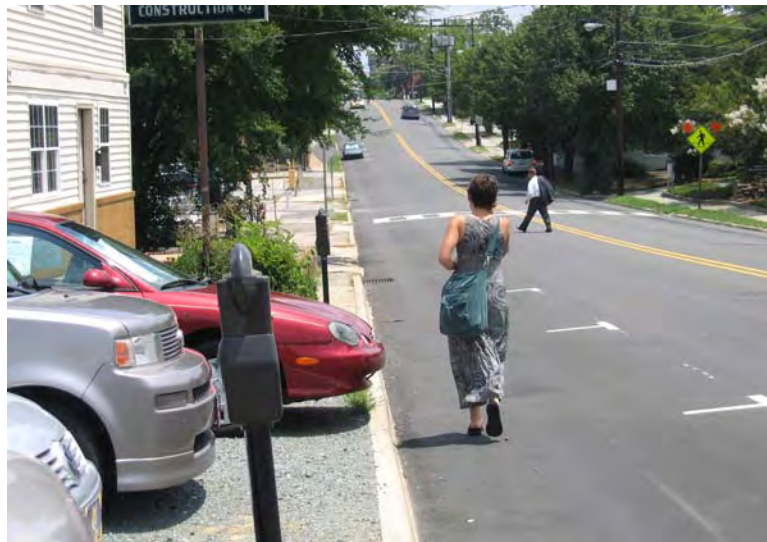
Figure 36. Pedestrians must enter the roadway to skirt parking meters and vehicles parked adjacent to Rosemary St. When the on-street spaces are occupied, pedestrians may have to walk in the middle of the traffic lane.
