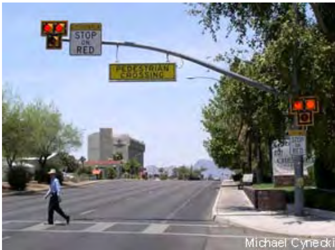
Figure 27. A HAWK signal provides a pedestrian-activated, stop-controlled crossing at midblock locations or other locations that do not warrant a regular traffic signal. (Photo by M. Cynecki)
