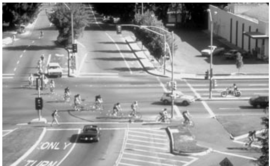
Pavement guide lines at signalized intersections can facilitate the movement of left-turning bicyclists.
