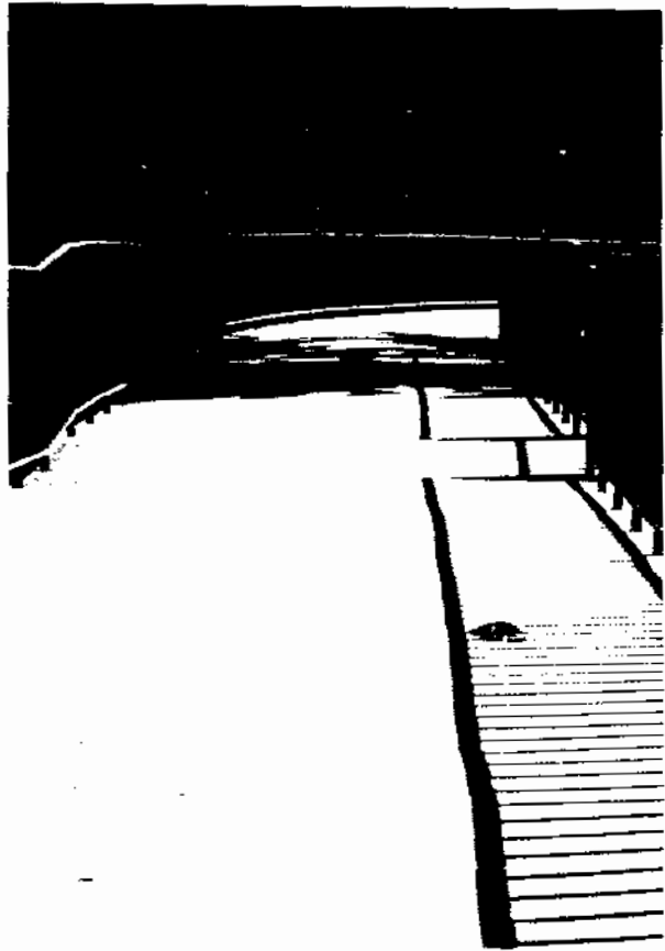
View of ramp showing level rest area partially up the grade
