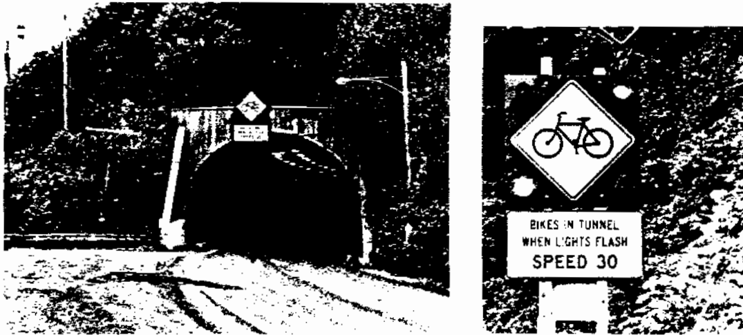
Figure 24. WARNING SIGN SYSTEM BIKE PRESENCE IN TUNNEL
