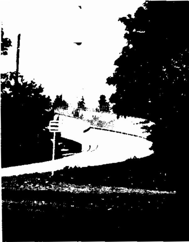
New ramp connecting bridge approach to ramp
