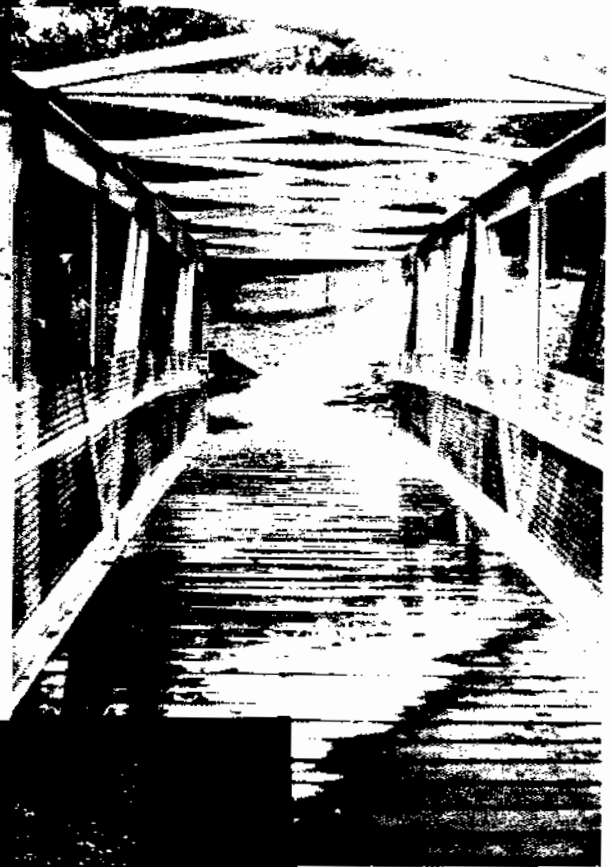
Bikeway bridge close-up
