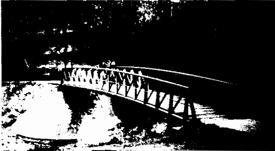
Bike/Pedestrian bridge connect pathway to culvert underpass
