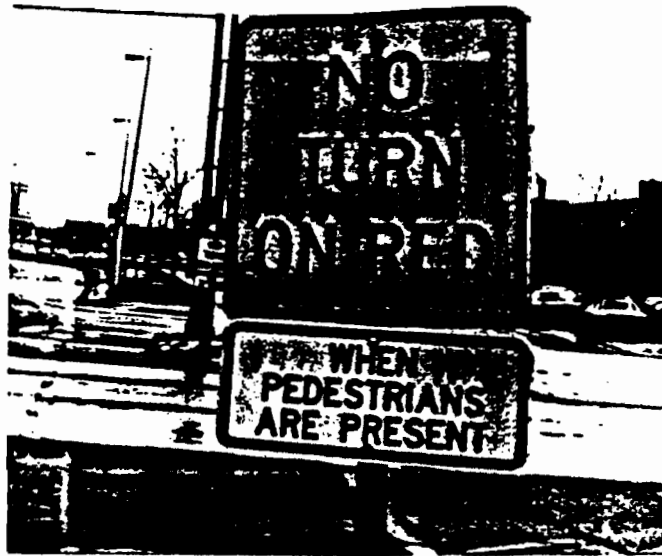
Countermeasure 3. NO TURN ON RED WHEN PEDESTRIANS ARE PRESENT sign
