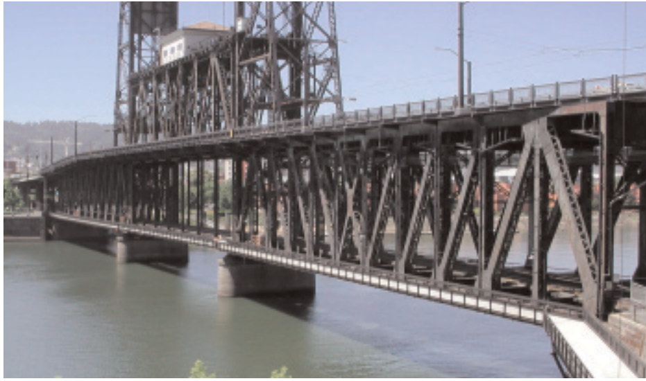
Steel Bridge Riverwalk. Portland, OR
