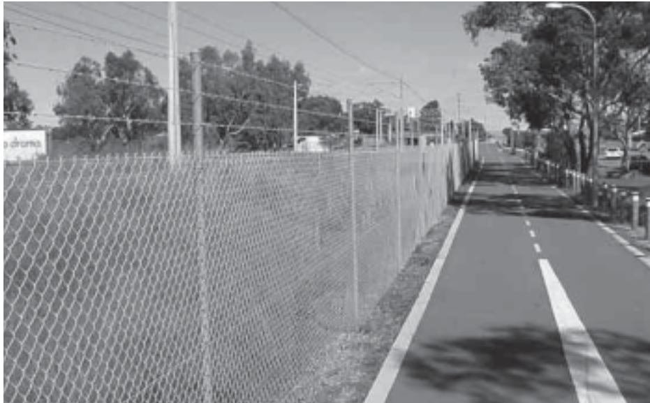
A section of RWT in Perth illustrates typical design and construction parameters, including 3 m (10 ft) wide asphalt path, set back from the adjacent rail line, and a 1.8 m (6 ft) chain mesh fence with three strands of barbed wire. Perth, Australia
