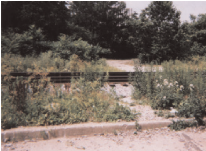
Current illegal crossing location over CSX tracks on Three Rivers Heritage Trail. Pittsburgh, PA
