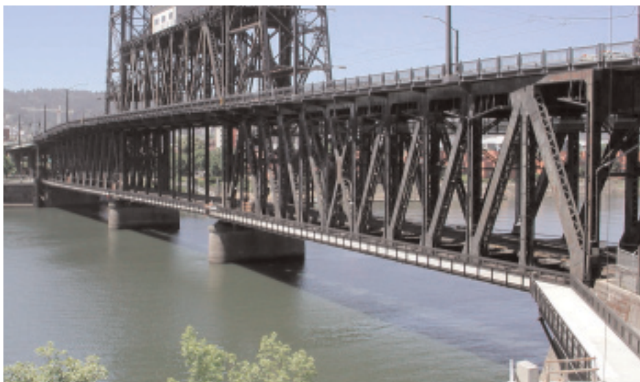
Steel Bridge Riverwalk. Portland, OR
