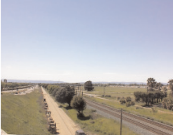
The Union Pacific Railroad planned track expansion led to a search for better alternatives. Davis, CA
