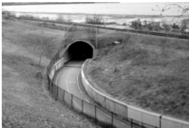
Undercrossing of Alaska Railroad Corporation tracks, Tony Knowles Coastal Rail Trail. Anchorage, AK
