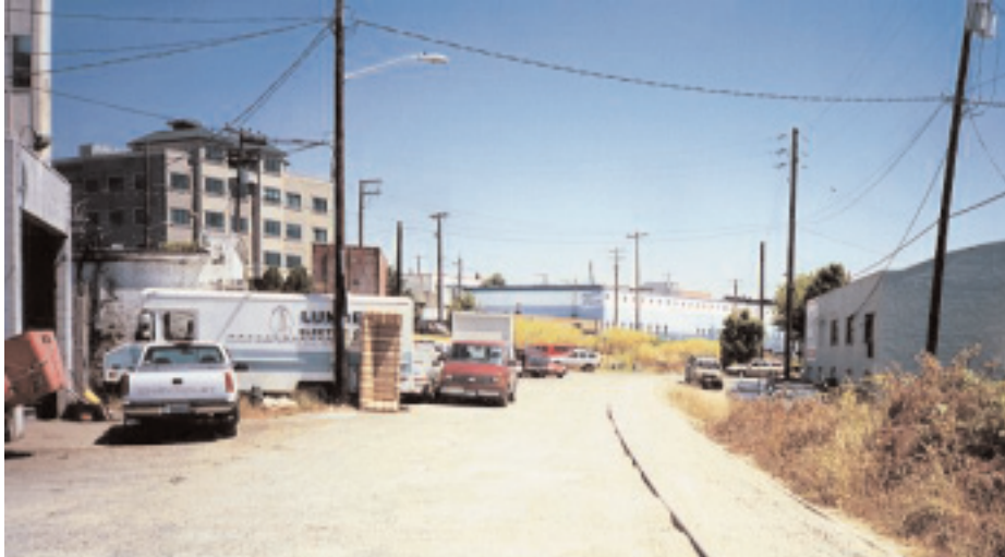
Planned future site of the Burke-Gilman Extension along the BTR tracks. Seattle, WA
