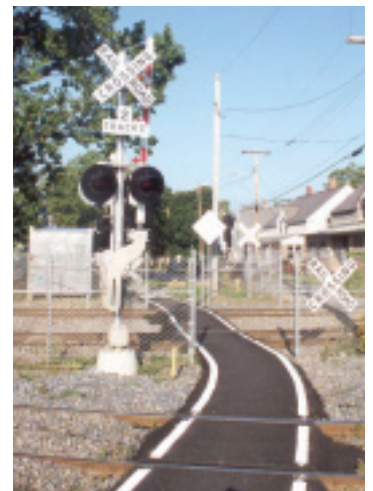
Dual track grade crossing. Burlington, VT
