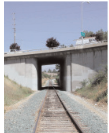
and must be rerouted in others. Cupertino, CA
