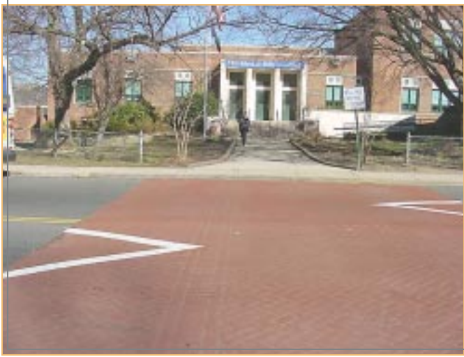
Speed table with stamped asphalt.
